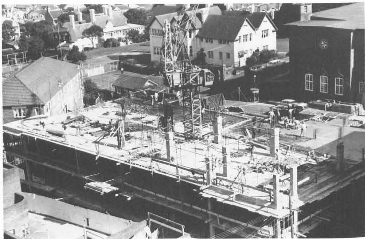
Above: Concreting the second floor of Benefactors on 22 May 1963. Photographed from the AMP Building.
